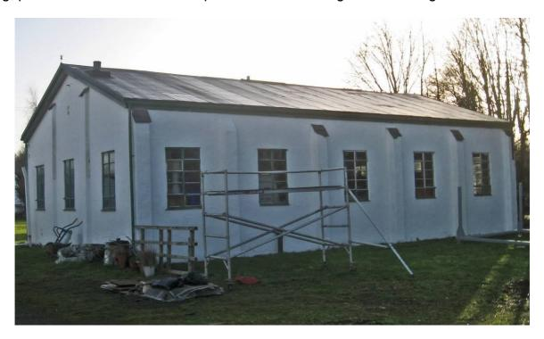
As can be seen from the photos the big difference is the windows fitted to 3 sides of the building and the height, what I have not shown is the floor and foundations, this building has them!! There is no water penetration at floor level unlike Bldg 28 and no condensation from the roof as it is a wooden roof covered in felt which is due for renewal in the spring.
