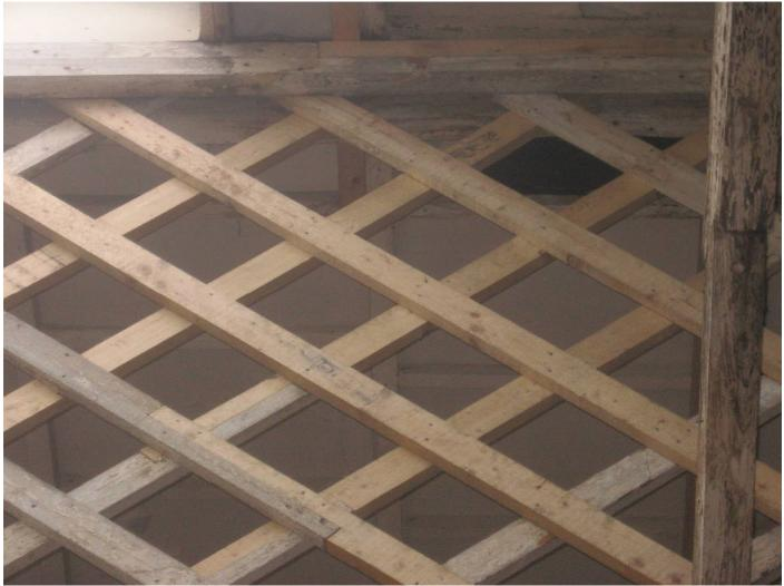
This is a close up of the worse trust and the last to be repaired, ravaged by wood worm you can see that in this area most of the wood had to be replaced. The repair does not include replacing the cement / asbestos roof panels but HPT believe for now it will be about 95% water tight.
